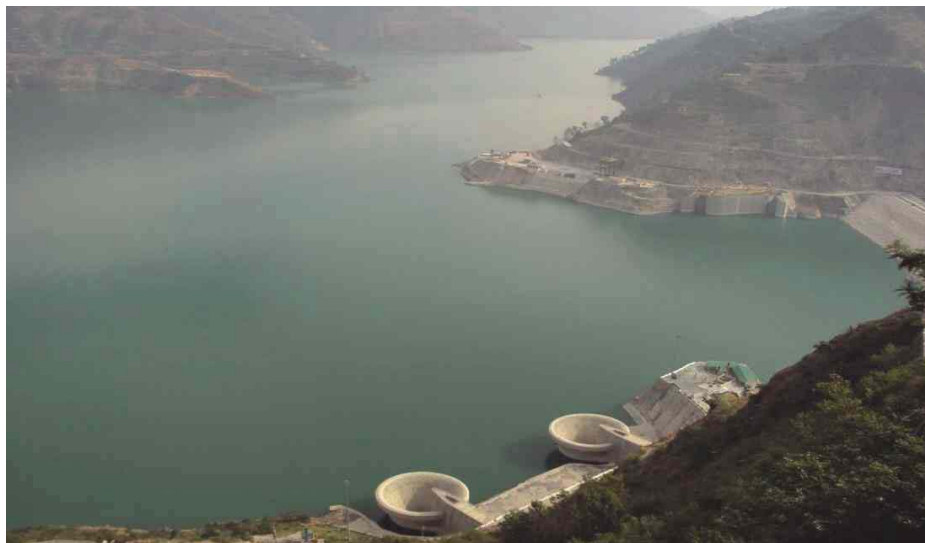
A View of Right Bank Shaft Spillway (Morning Glory) of Tehri Dam Site
