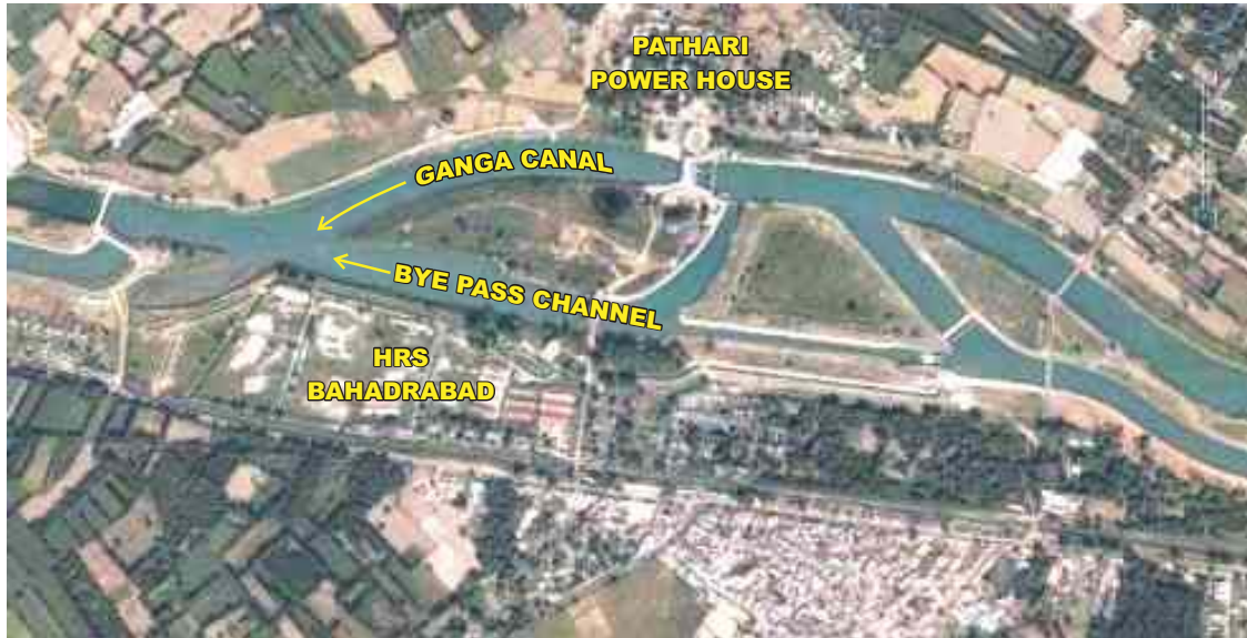
A Panoramic View of Hydraulic Research Station, Bahadradab from Google Earth
